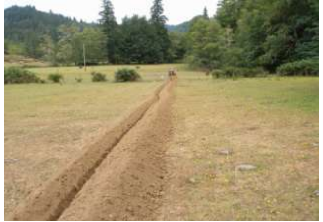
More Trenching Work
