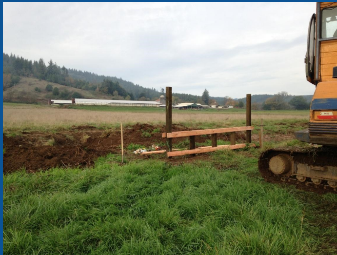
Project Implementation: construction of 'elk-braces' for wildlife stream crossings, Fall, 2016
