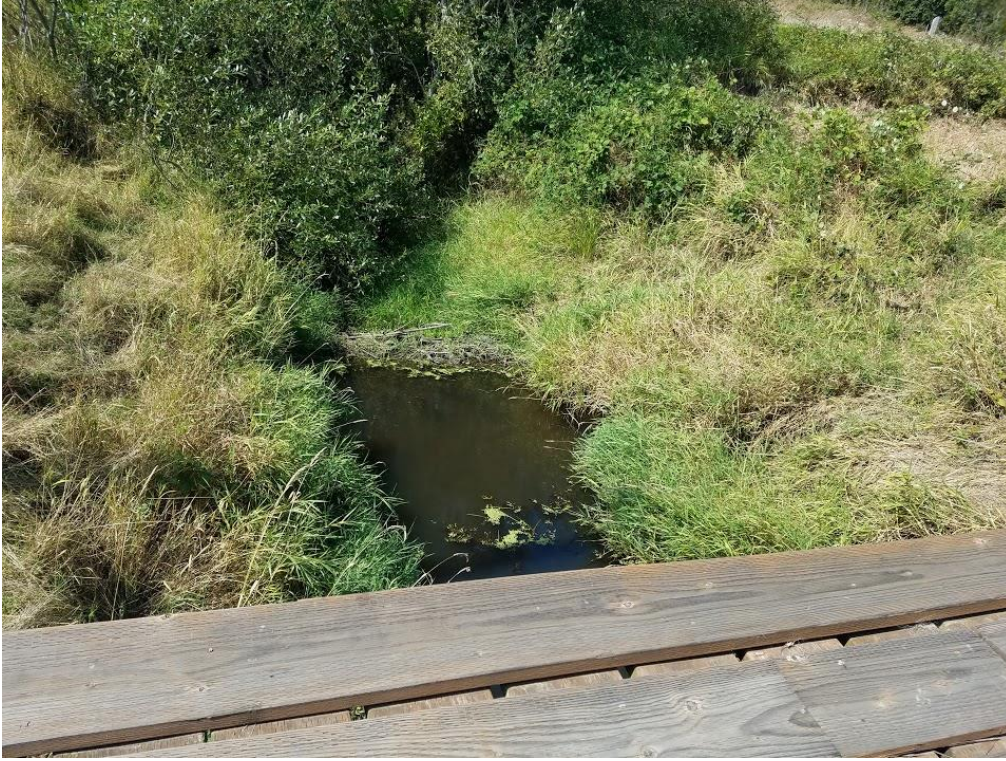
Figure 11. Site E7 is at a bridge over Bear Creek on the Tigard property.
