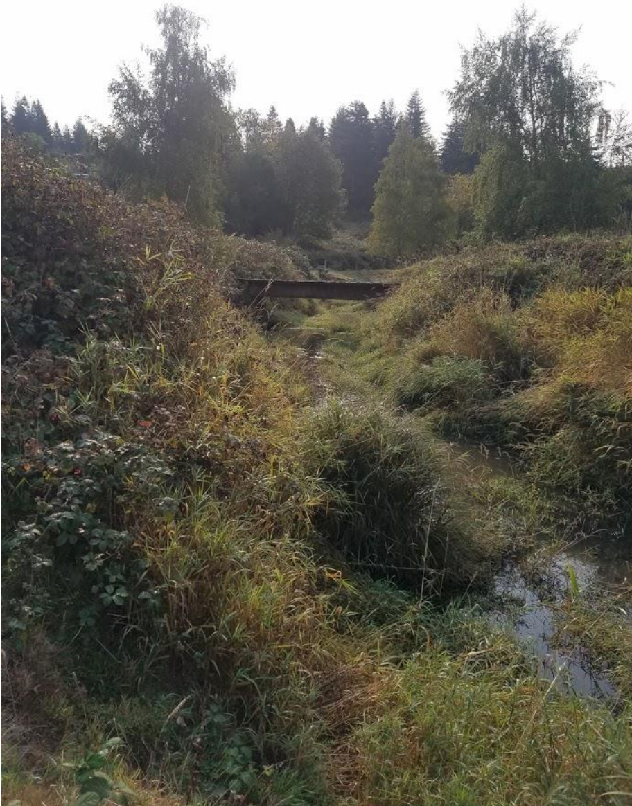
Figure 12. Site E8 is at a bridge over Bear Creek on the Aitchison property.
