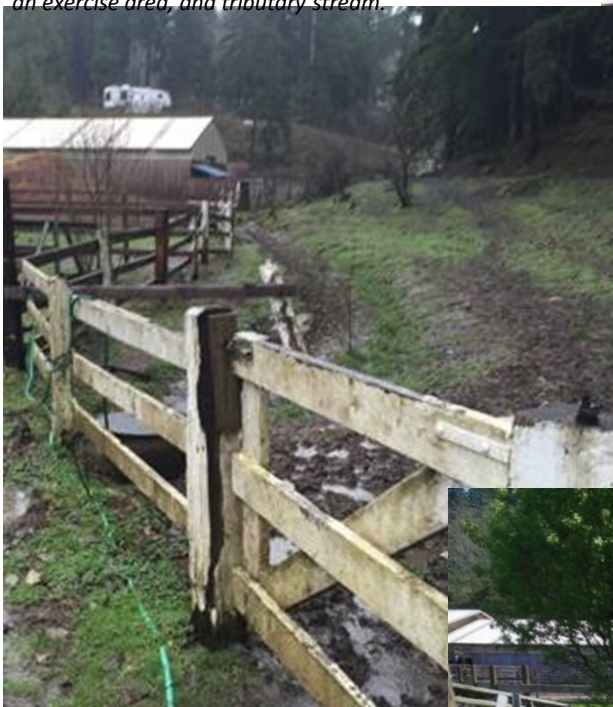
(Below) Initial site visit, December 2015 shows original condition of the small hillside pasture which was being used as an exercise area, and tributary stream.
