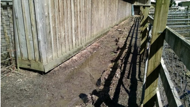
Main Barn, adjacent drainage: BEFORE (6-14-2017)
