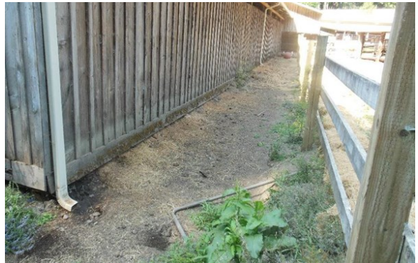
Main Barn, adjacent drainage: AFTER (8-8-2018)
