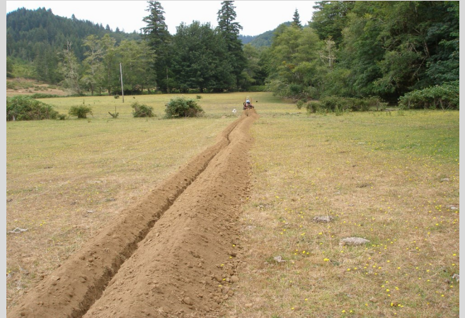
Trench work continues
