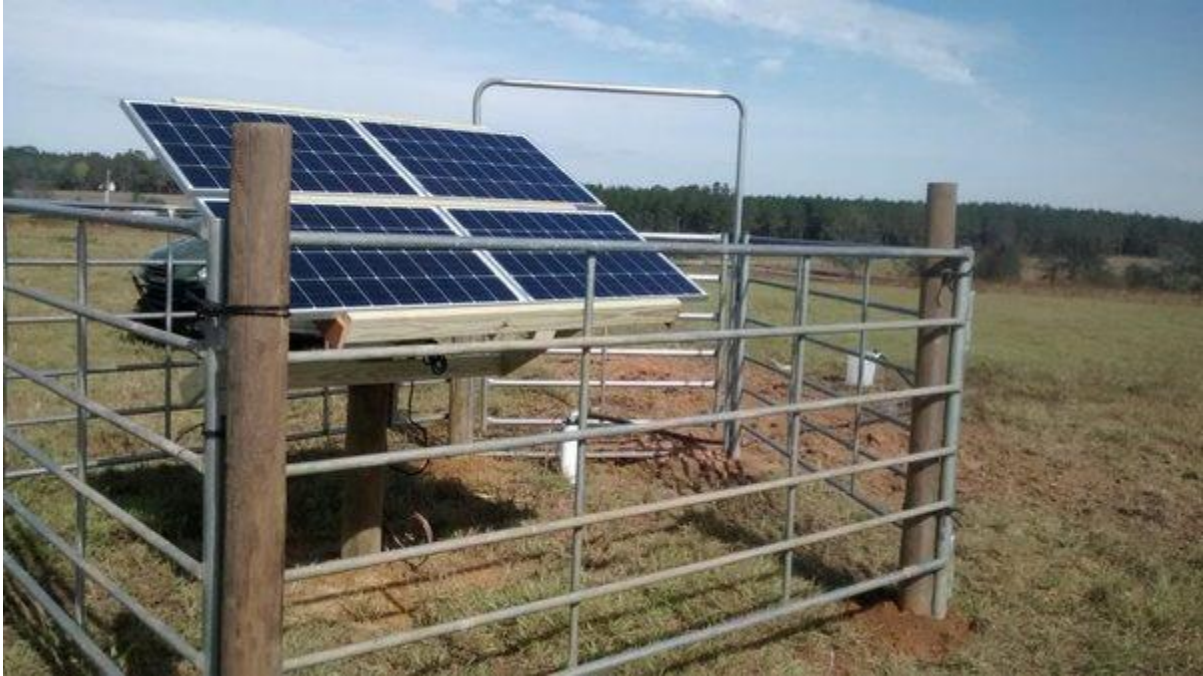
Figure 1. Example of Solar Panel Installation with Protective Fencing
