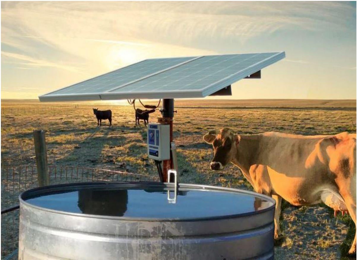
Figure 2. Example of Solar Panel Installation with Watering Trough on a Heavy Use Area Protection
