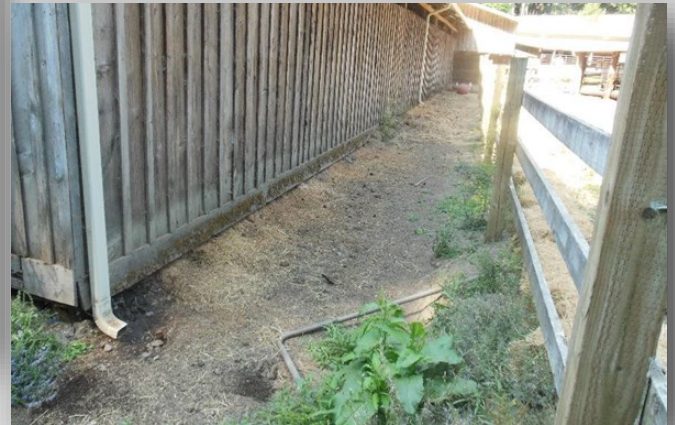
Main Barn, adjacent drainage: AFTER (8-8-2018)
