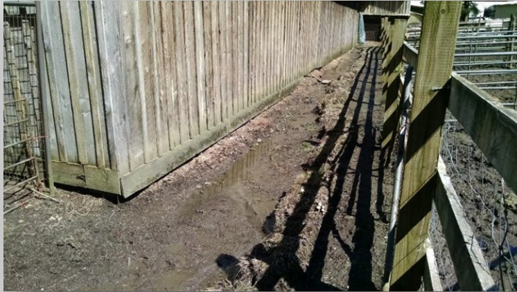
Main Barn, adjacent drainage: BEFORE (6-14-2017)
