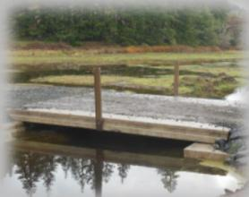
*Collapsing culvert replaced with concrete slab bridge at a livestock crossing*
